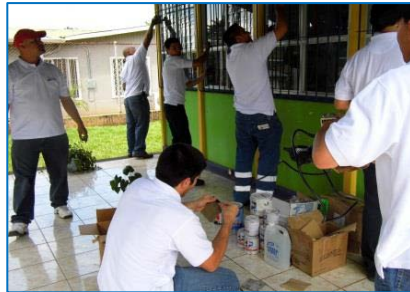
Ruta 27 employees in San Pablo School
